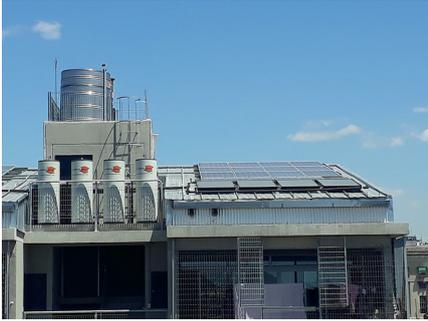
A total of 174 solar panels and 55 solar-powered water heaters were installed on the rooftops of the new social housing complex in Villa 31, in the Argentine capital. Each water heater has a capacity of 300 liters and supplies two homes, based on the estimate of an average of three people per apartment, who use 50 litres of hot water a day. Credit: Daniel Gutman/IPS
